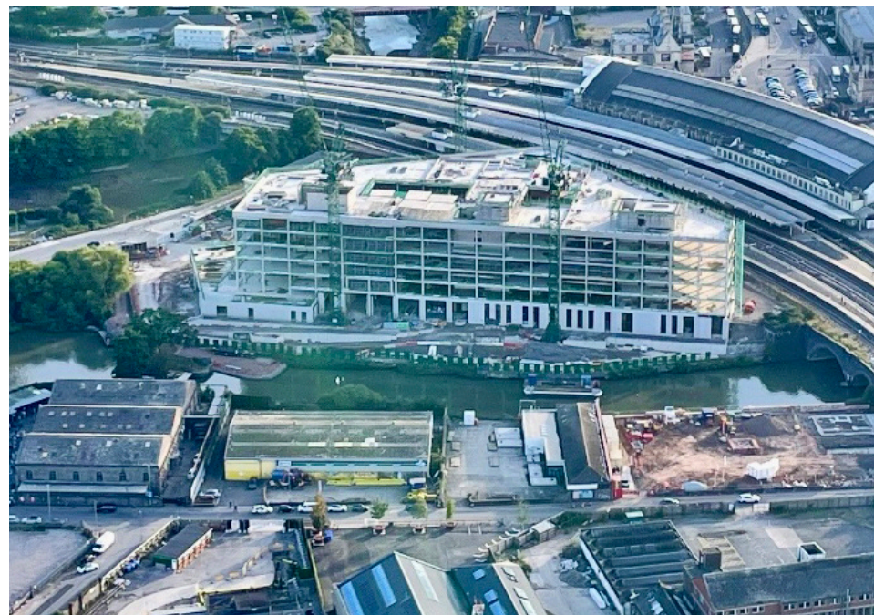
Emerging TQEC Phase 1 - Site Progress
