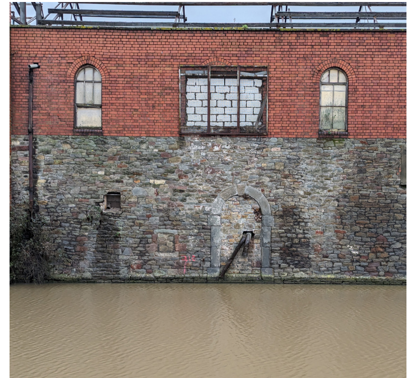
Existing Rubble and Brick Structures
